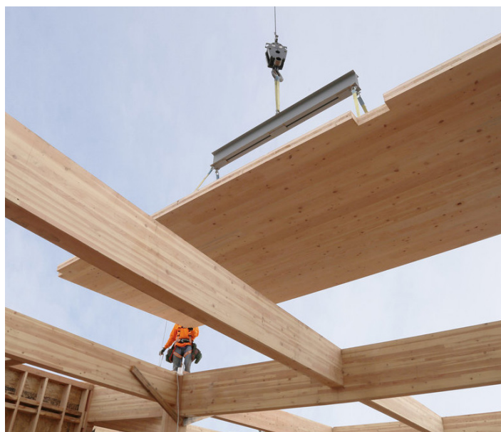
Construction of Albina Yard | Source: Lever Architecture
